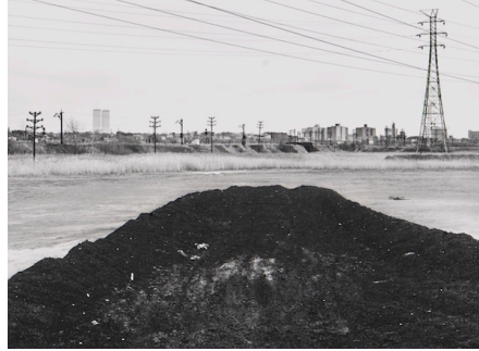
Hudson Generating Station, Jersey City, 1979
